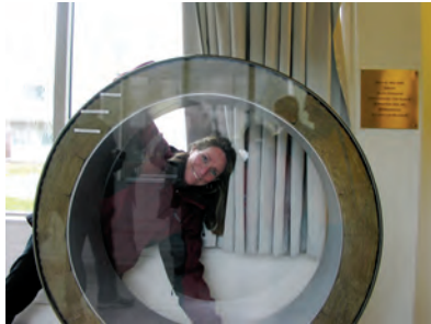
Julie B-G sizing up pipes used for moving hydrothermal waters during a site visit with the ICDP in April 2007.
