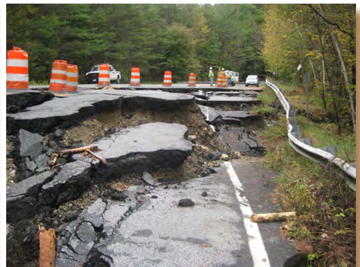
Pictures of some of the damage from Tropical Storm Irene along Route 2 in northwestern Massachusetts. Left: Translational debris slide along sheeting joints oriented 284^\circ dipping 38-40^\circ . Right: Rotational slide that moved along a layer of lacustrine sediments 5 to 6 m below the surface that were noted by Joe Hartshorn in earlier mapping of the Rowe quadrangle (Chidester et al., 1967)
